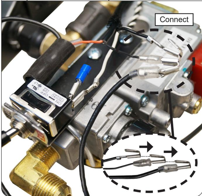
Put insulation on new connection
