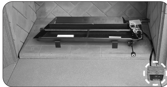
Fig. 16-2 Place heat shield (if applicable)
