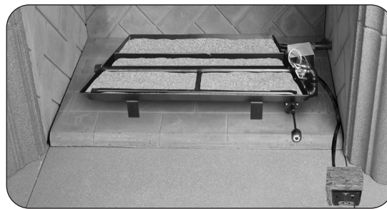
Fig. 22-1 Place sand/vermiculite
